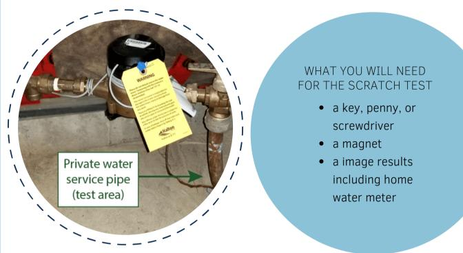
First, you will need to locate your water meter, usually found in your basement. As seen above, your service line will feed into this. This is where you will perform the scratch test.
